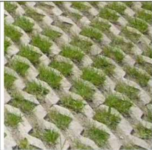
Concrete grass slabs Graskeien
